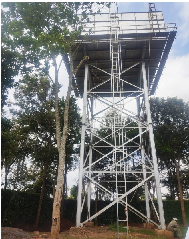
Tetu Elevated Tank construction ongoing.
