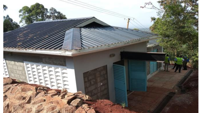
Generator room & Pump station at Mathari Twin Tank.
