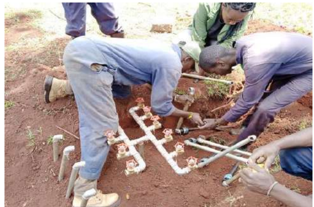
Meter separation at Kiganjo police college to enable individual connections to police quarters.
