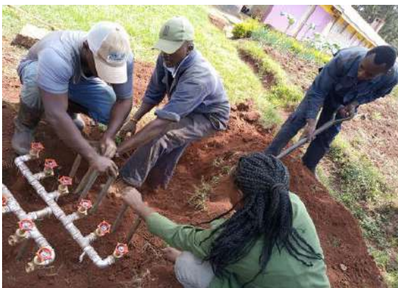
Meter separation at Kiganjo police college to enable individual connections to police quarters.
