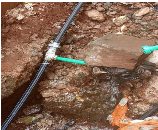
Examples of illegal water connections nabbed by the Security and Investigations section during the month of January 2022
