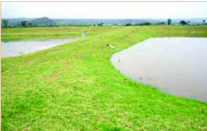
Stabilization ponds for sewage treatment.
