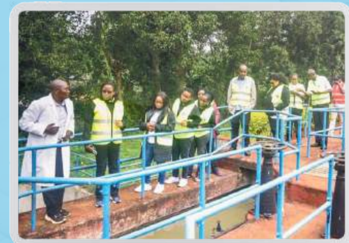
Board members at the Kangemi sewer treatment plant during a board inspection tour.
