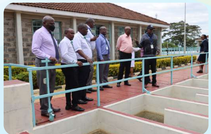
TWWDA Board Members tour Kamakwa Treatment Plant
